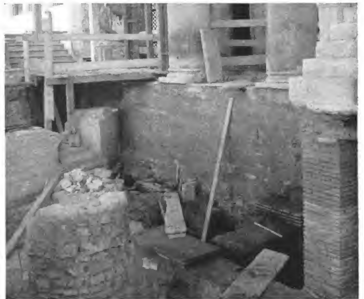
Fig. 21 — S. Lorenzo f.l.m. West basilica, south colonnade foundation wall, and East basilica, apse H, 1949 (Photo: Soprintendenza ai monumenti).
